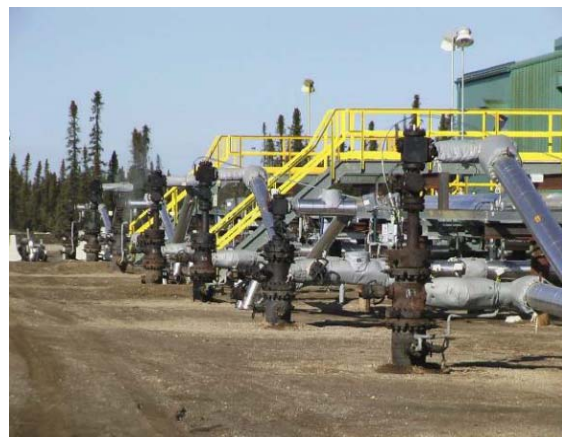
Figure 3 Halliburton SAGD wellhead surface layout
